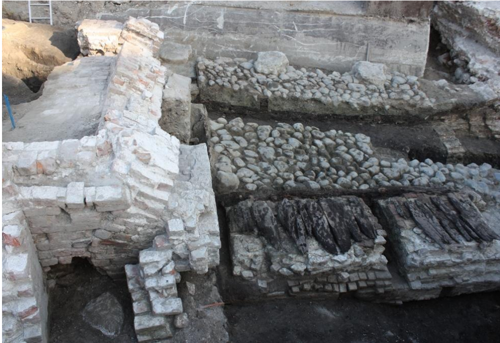
Figure 139 The upper (later) part of the head race within the former bridge arch, where it would have entered the mill. Seen from southeast
