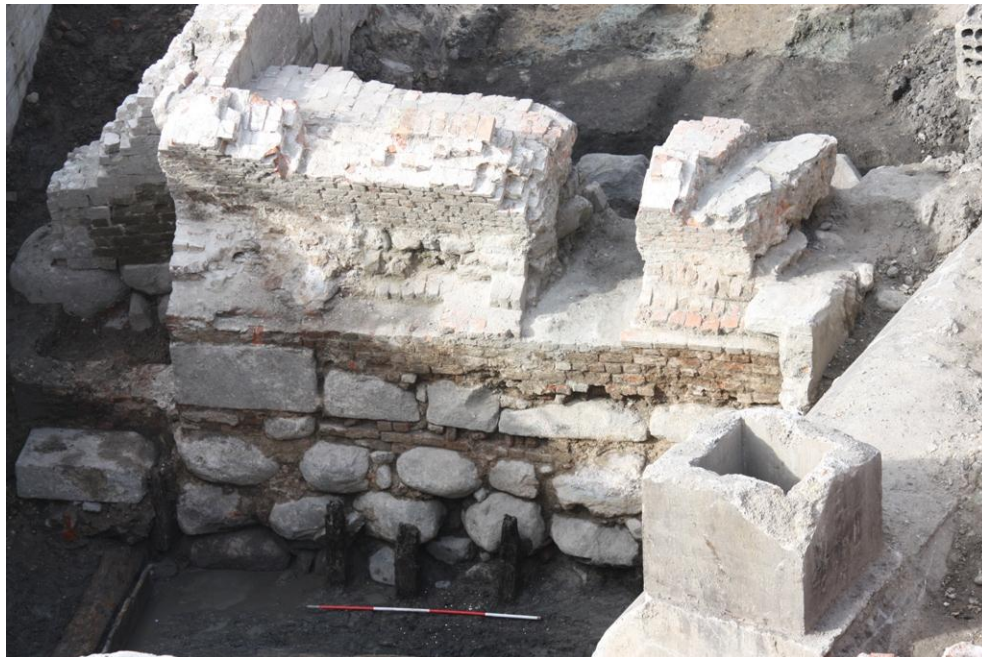
Figure 127 The western side of the bridge arch, with foundation boulders and timber uprights visible
