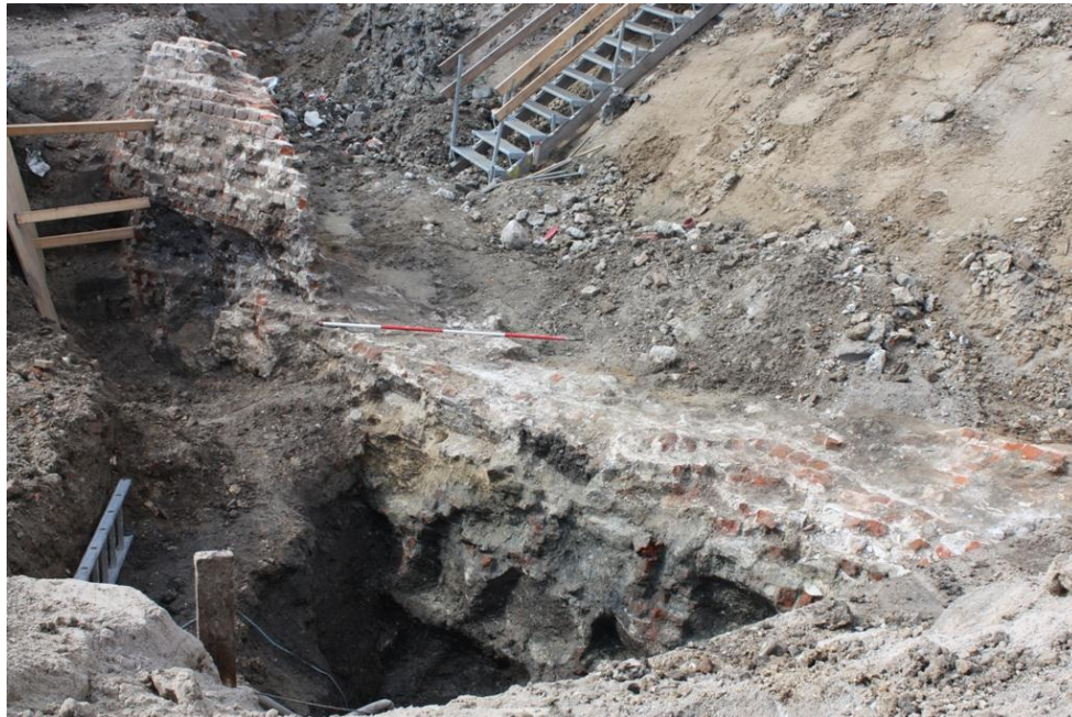
Figure 130 The robbed-out face of the bastion
