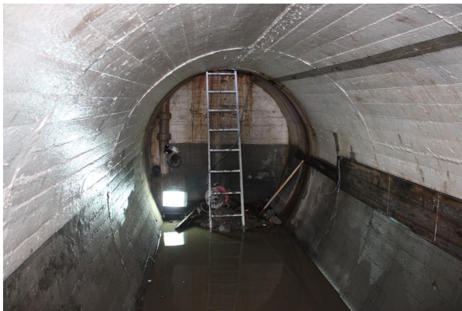
Figure 135 The interior of the shelter in Area 2B. Note the wooden panel and wires to the right, and the ceramic pipe in the corner
