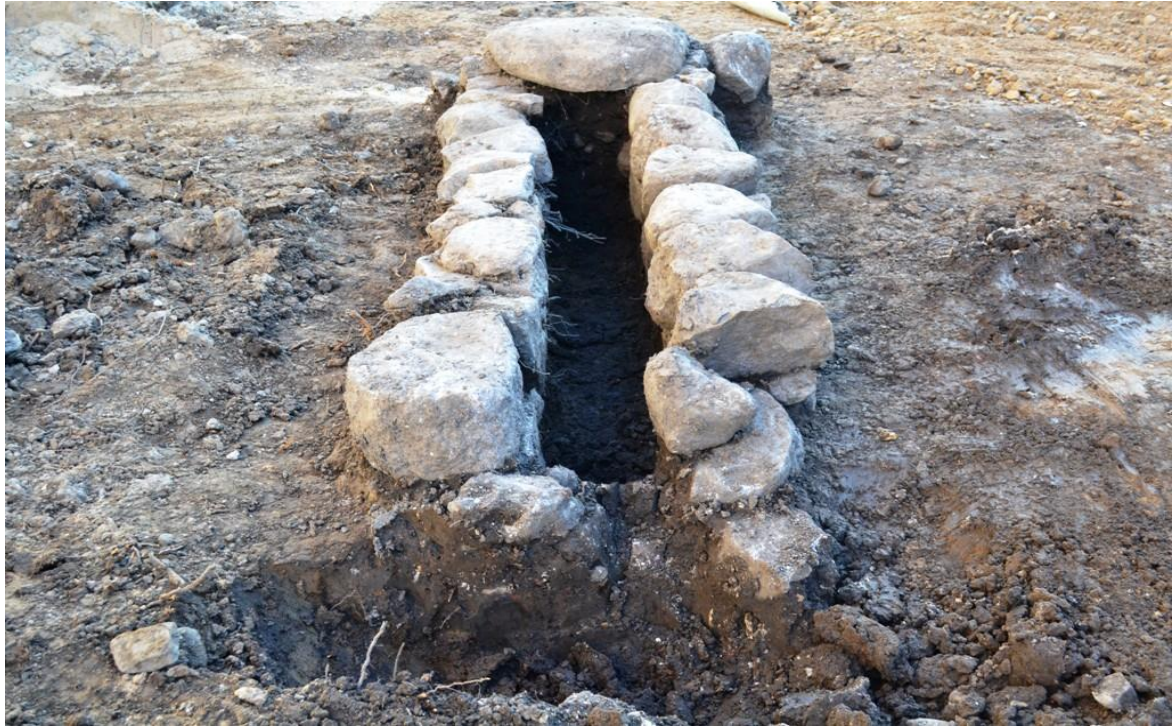
Figure 25 Skjolds Plads. 19 th century stone culvert.
